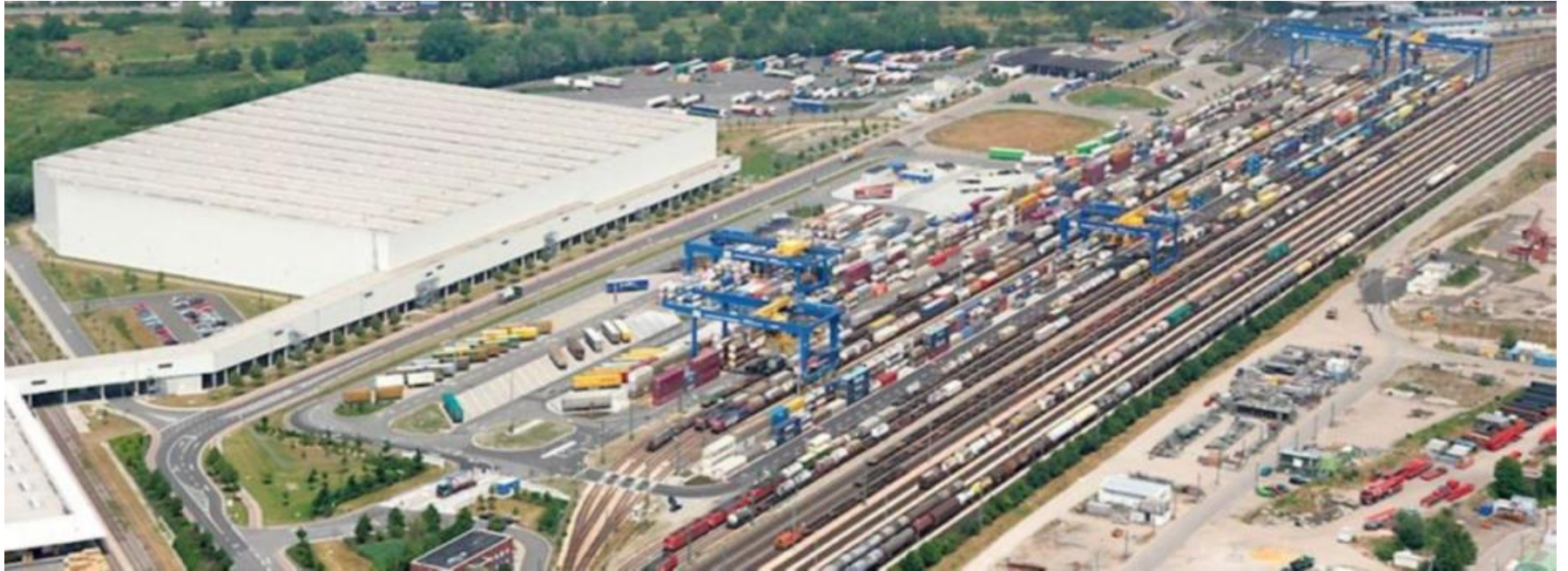
Multimodal terminal in Bucharest (road - railway)
